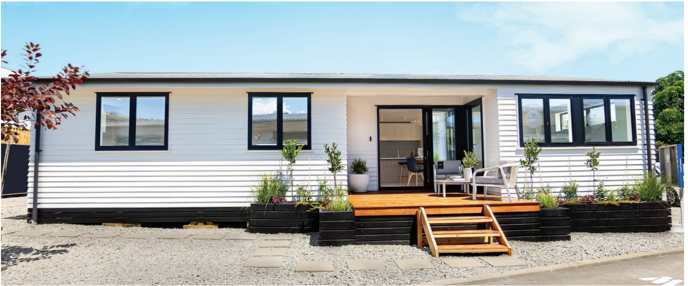
Kāinga Ora house, One Tree Hill Trade Academy renovation, Auckland
